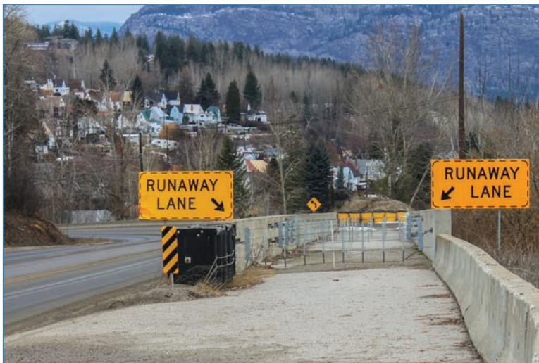
This type of runaway lane relies on a cable netting system and a rock bed to slow down the truck on either a horizontal or descending grade. You'll need to be accurate with your entry as there are concrete walls on both sides of this
